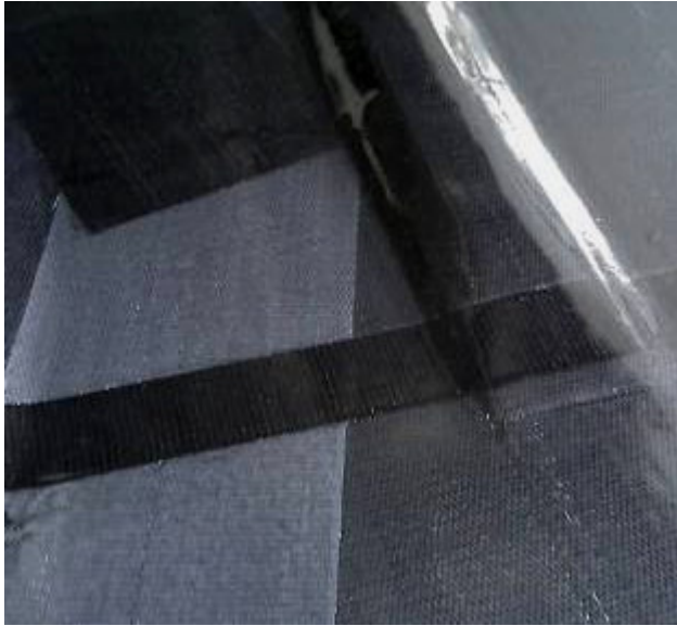
Carbon fiber interior laminates for strength and stiffness, finished clear
